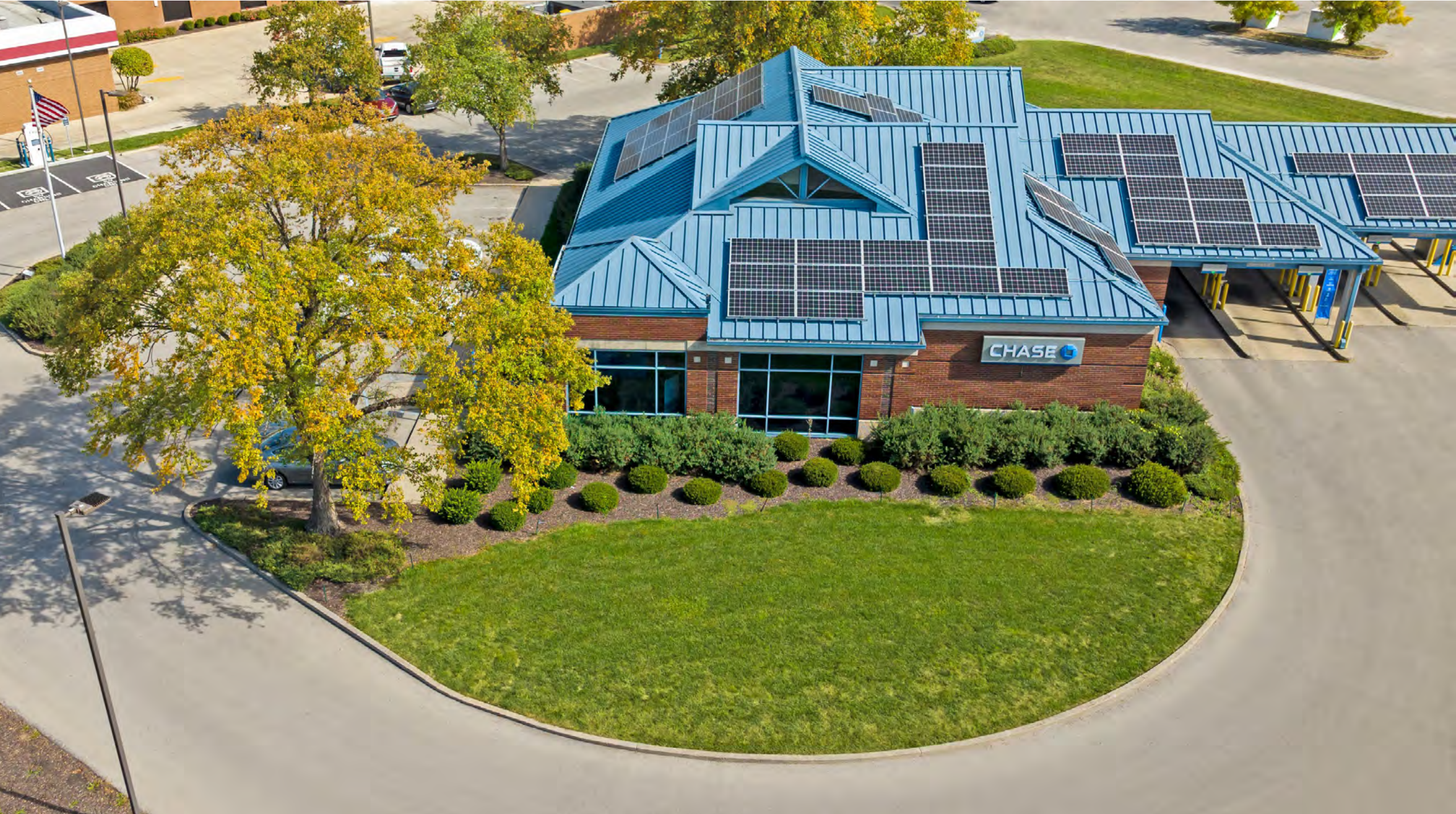
The Firm continues to expand on-site solar power at our corporate office buildings and retail branches across the U.S. Pictured: Carmel, Indiana. Image courtesy of EVgo.
