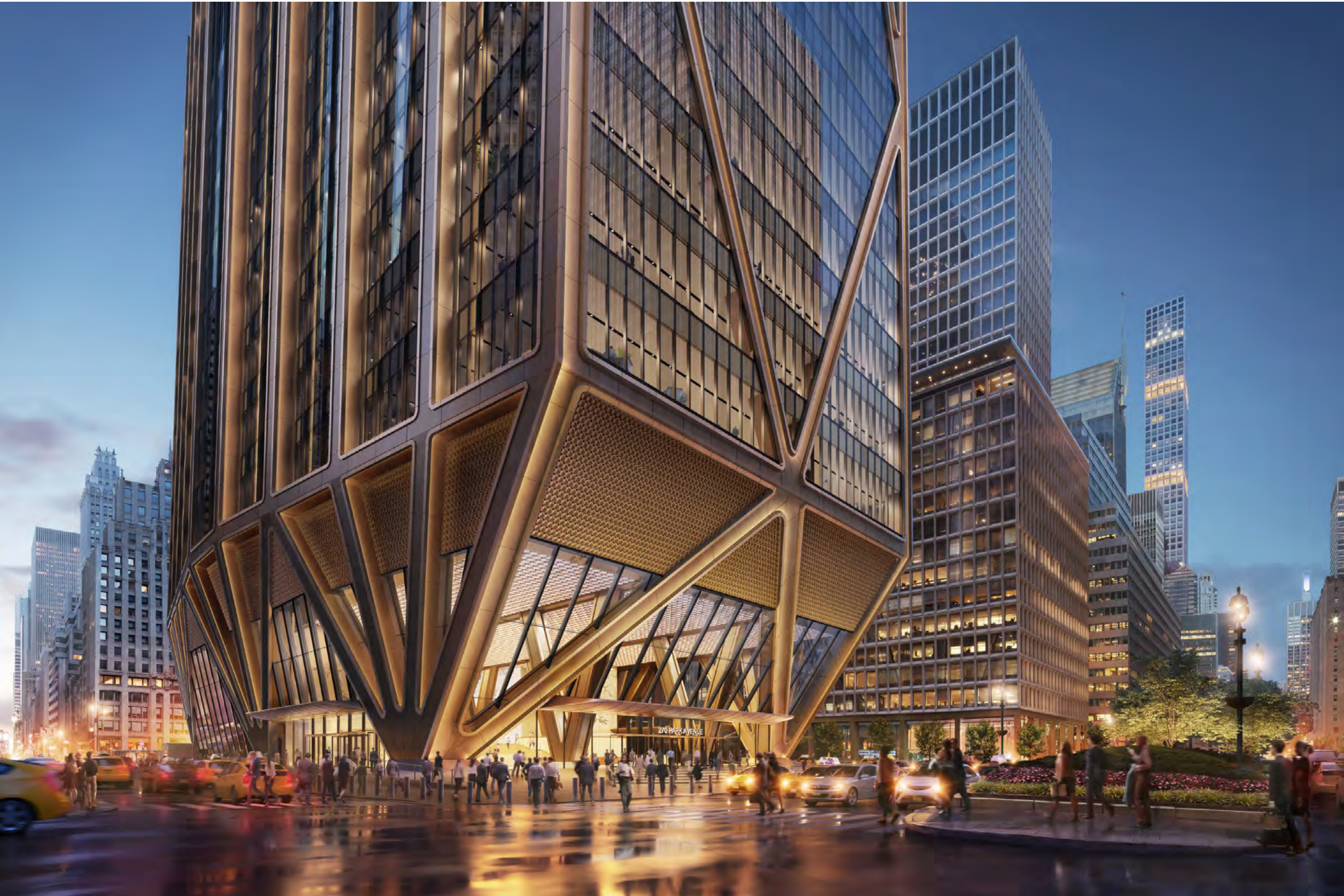
The Firm's new headquarters is expected to be Manhattan's first all-electric tower. Image courtesy of DBOX / Foster + Partners.
